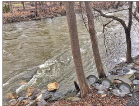
Concrete sculpted flowforms transform water from a Main Street storm drain that releases into the Housatonic River Walk in Great Barrington
